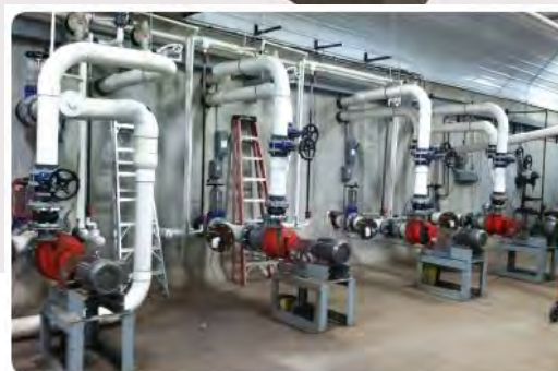
The technology at work in the biodigestion pilot plant
